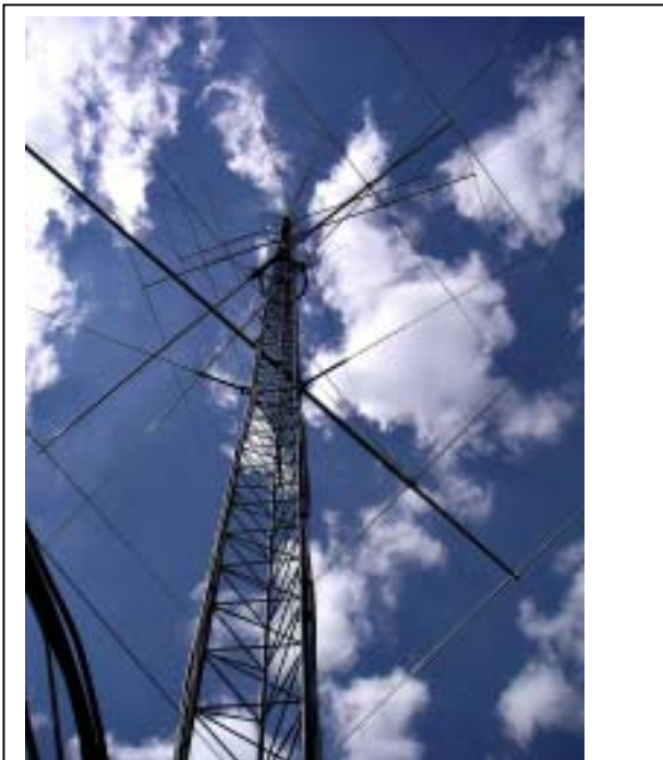
This is the 180 foot tower that holds the 40 meter beams. That is a 10 meter antenna at the top. "There's no meters like ten meters!" (Tower photo, shot from base, looking up)
