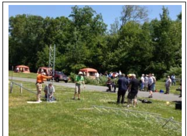
Beam team installs tower in foreground. Site teams practice site assembly in background.
