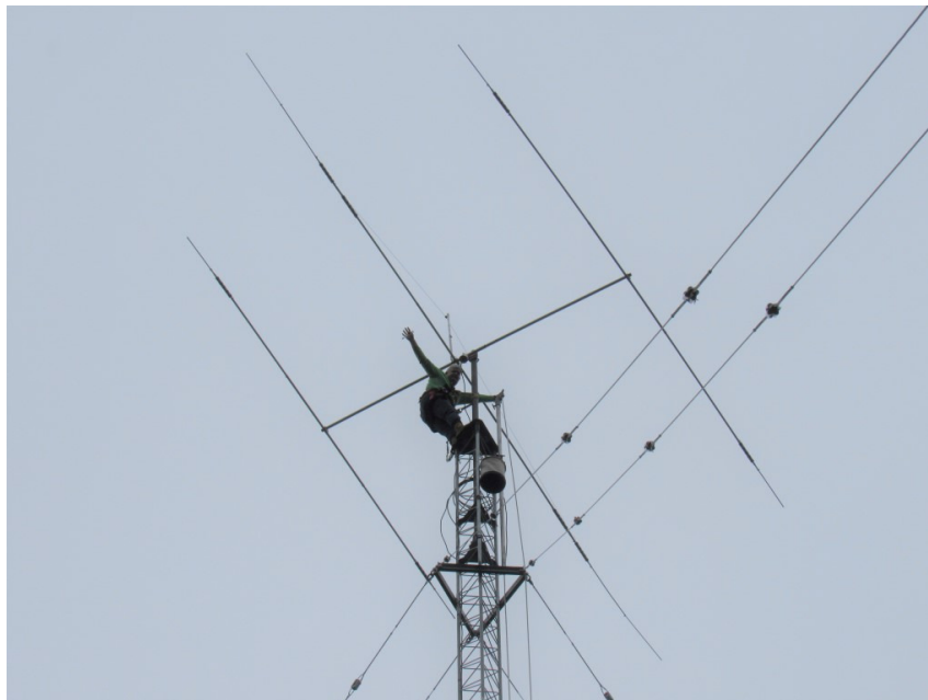
N1RR Rohn 55G 130ft tower in Seekonk, MA, First permanent antenna A3WS+30M up 139ft. Thanks to Randy-K5ZD and Jim-N1NK for their help on antenna. Photo credit: Jim Spears-N1NK
