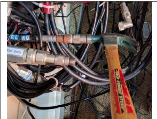
Photo 8: Take the barrel from the PL-259 you just sacrificed, screw it onto the barrel (to avoid damaging the barrel by hammer blows) and “persuade” the whole connector into place. You will be glad that the Penetrox™ has some lubricant in it.
