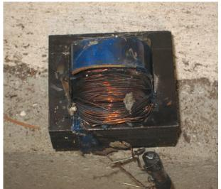
it is a good dielectric. The lightning discharge, seeking ground, had jumped from the stricken tree's roots (full of water and thus electrically conductive) to the multi-wire cable that passed through this hand-hole on its way from the irrigation system controller in my house, to the system's several valve-solenoids.
