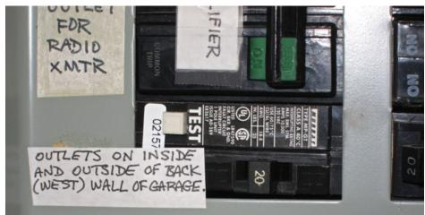
Unfortunately, the shortest electrically-conducting path to ground was not the big thick cable that delivered up to 60 A at 240 VAC to this sub-panel from the main, 200-A, panel or "load center" at the utility service entrance in the basement, halfway to the opposite end of my house.
