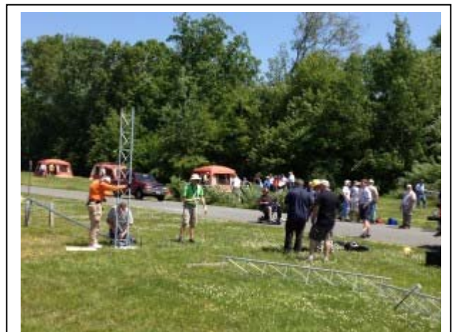
Beam team installs tower in foreground. Site teams practice site assembly in background.
