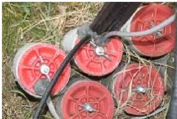
Sealing the pipe ends is done with 4-inch plumbers water pressure plugs which are available at home depot or other plumbing supply. I notch the plug to allow for the coax then seal it all with electrician outdoor seal (commonly called monkey s\_\_t).
