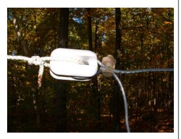
My 160 wire is 10 AWG, and the photo shows how I keep the wire from sliding in the insulator where it goes from vertical to horizontal.
