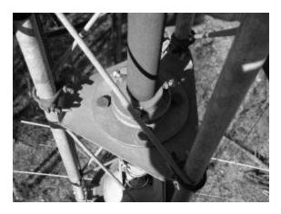
Figure 2 Detail view of lower thrust bearing mounted on standard rotor shelf. Note the Z-braces were cut to allow shelf to be mounted at this spot in the tower section
